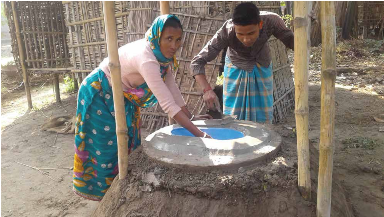
Photo 44: Participants building toilet for better sanitation through support from SWARP (ESDO-Water Aid Bangladesh)
